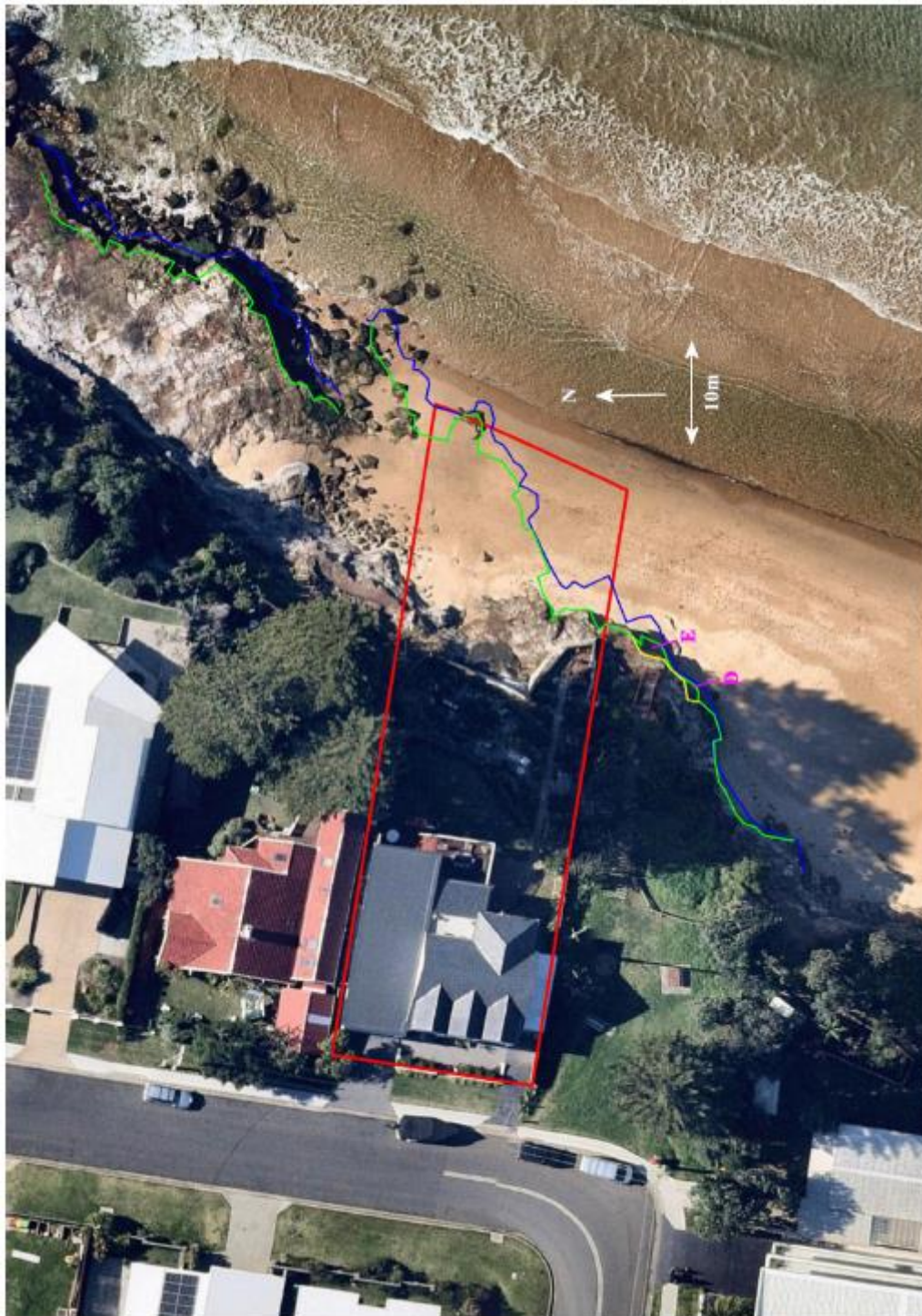
Aerial photograph of 1 Craig Street Thirroul on 26 June 2020, with seaward edge of cliffline delineated in yellow (12 January 2010 cliffline in blue, and 18 March 2020 cliffline in green)
