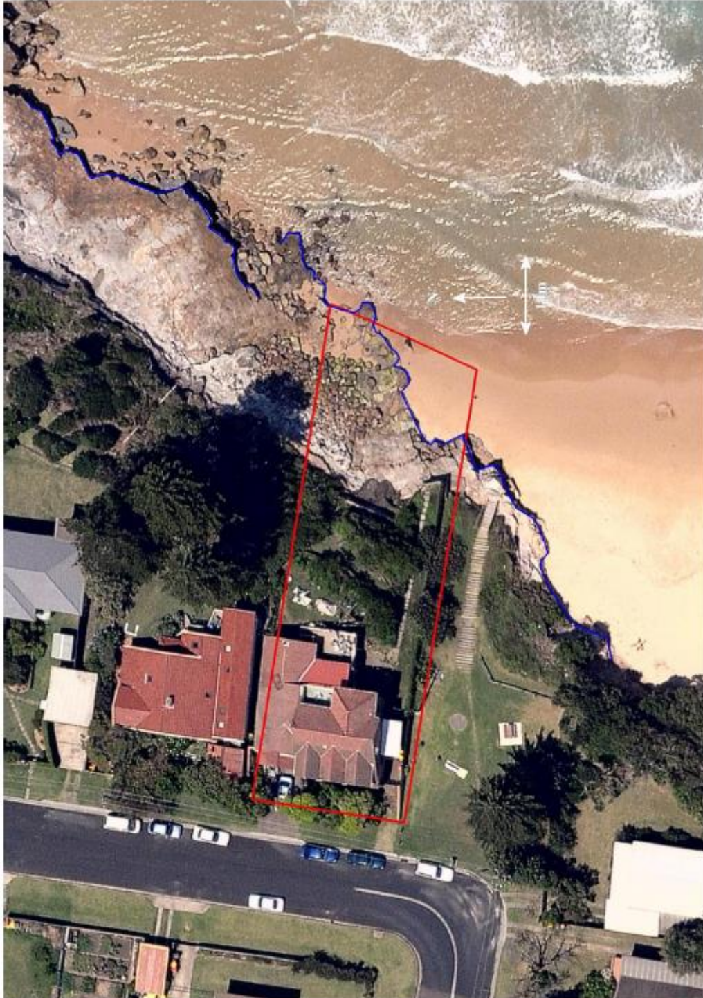
Aerial photograph of 1 Craig Street Thirroul on 12 January 2010, with seaward edge of cliffline delineated in blue
